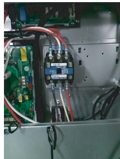
* cables connection between constant compressor and magnetic switch
