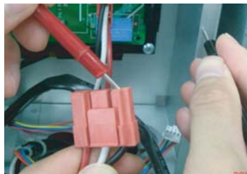
Measuring insulation resistance between fan terminal & chassis
