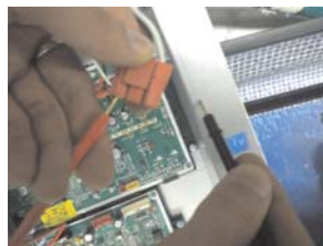
Measuring insulation resistance between fan terminal & chassis
