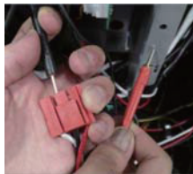
Measuring insulation resistance between fan terminal & chassis
