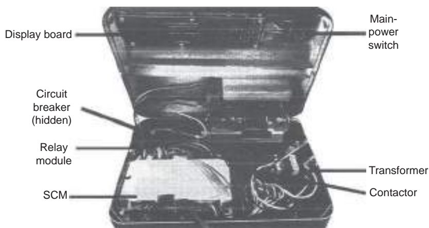
FIGURE 12.5 Electrical section. ( Carrier )
